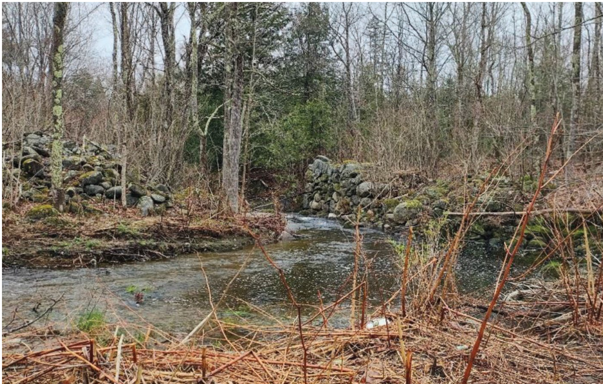
Exhibit 9. Remnant bridge abutment, northeast corner of property. (Photo: Haley Ward, Inc.)
